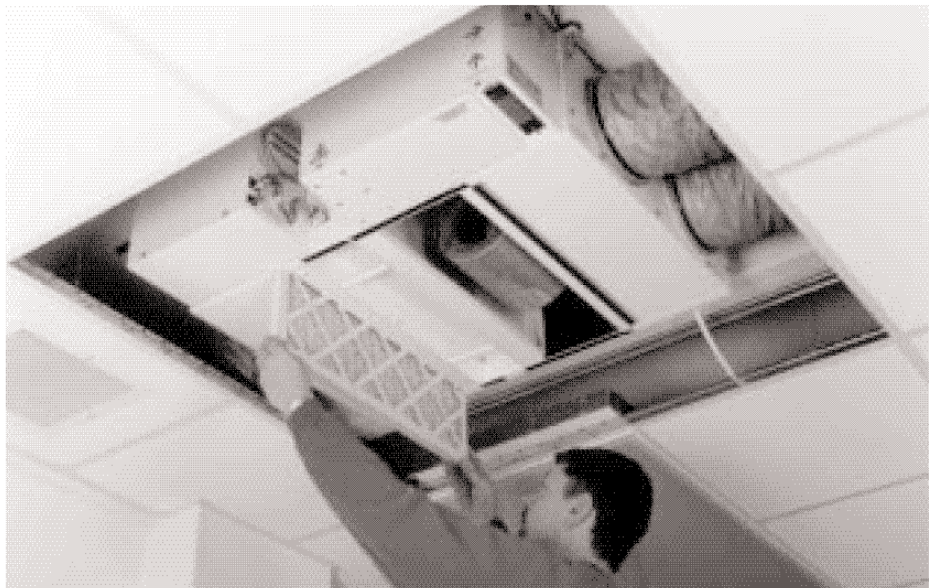
▲ The detachable bottom cover gives access to the antibacterial air filter, humidification cassette and fan
